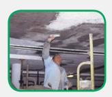
MEADOW-CRETE GPS is a one-component, trowel applied or pneumatically applied (wet process), migrating-corrosion-inhibitor enhanced, polymer-modified, shrinkage-compensated, fiber reinforced, micro silica enhanced, cementitious repair mortar for horizontal, vertical and overhead applications from 1/4" to 4" in depth.
