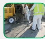
FUTURA-45 EXTENDED is a pre-extended version of the standard FUTURA-45 containing 3/8" nominal size aggregate that will not promote alkali-silica reaction (ASR). To ensure long-term repairs, the aggregate is designed and tested to prevent decreased product performance that a poor jobsite aggregate may cause.
