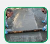
FUTURA-15 EXTENDED is a pre-extended repair mortar containing 3/8" nominal size aggregate that will not promote alkali-silica reaction (ASR). To ensure long-term repairs, it is designed and tested to prevent decreased product performance that a poor jobsite aggregate may cause.
